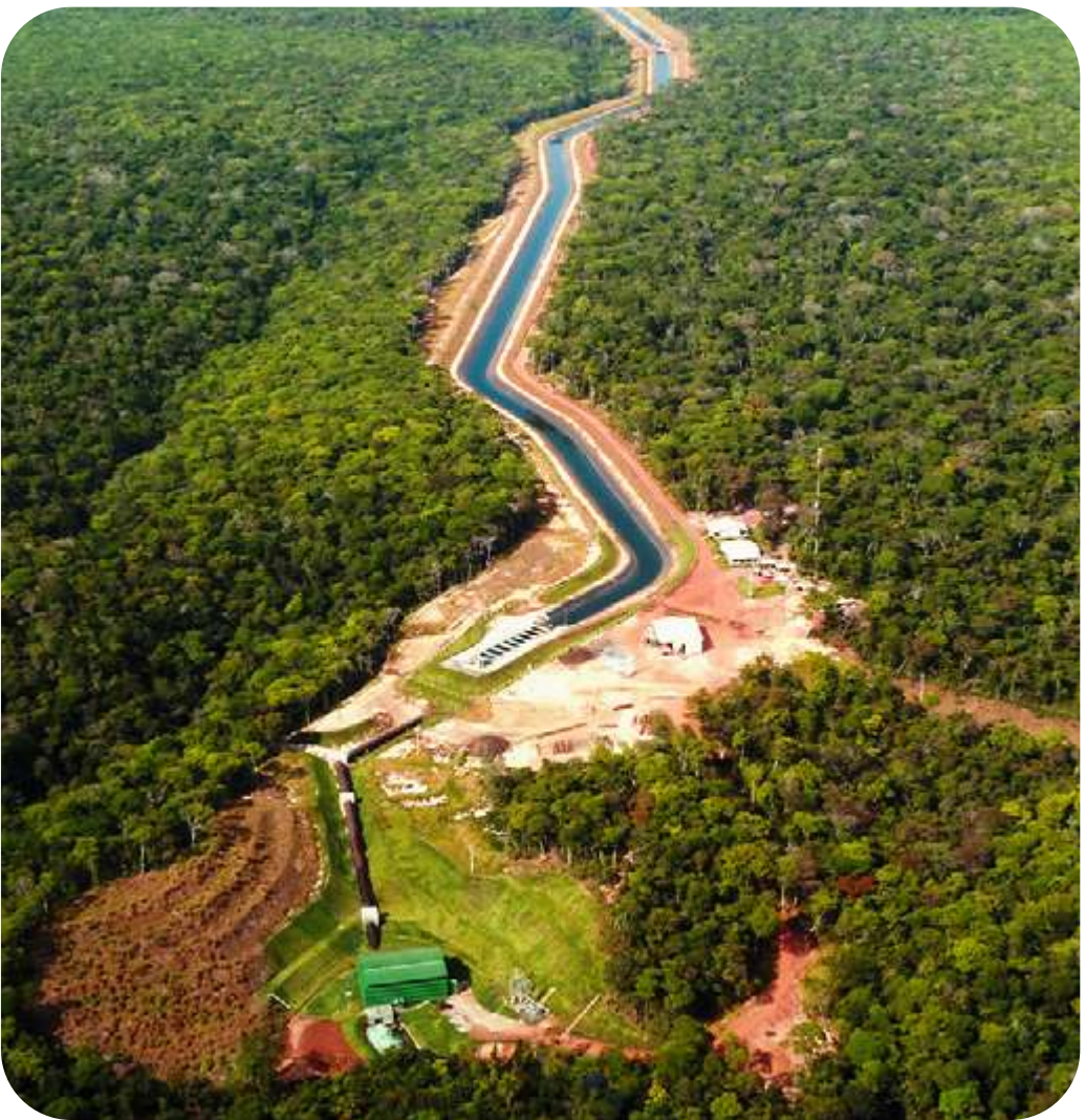
Água Quente Small Hydropower Plant (CGH) Sapezal (MT)
